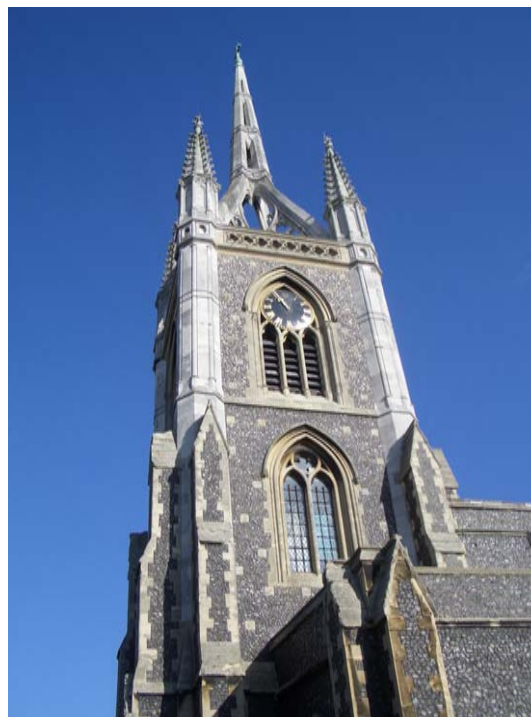
Picture 4.1.6 St. Mary of Charity, parish church of Faversham
